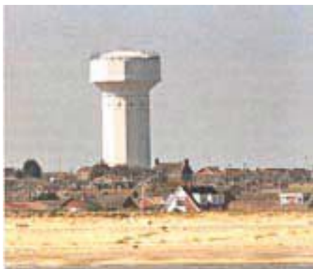
Caister water tower
