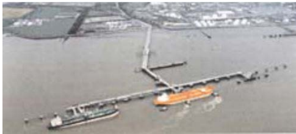
Immingham Oil Terminal
