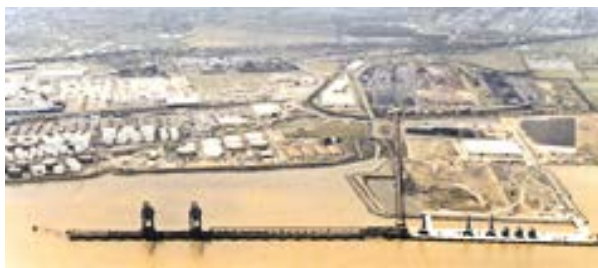
Immingham Bulk Terminal
