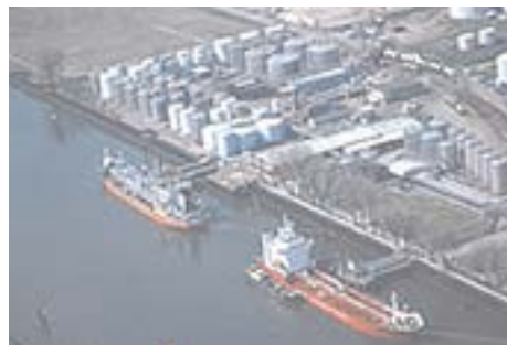
Hamburg Oil Terminal
