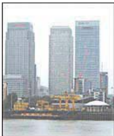
Canary Wharf Tower (center)
