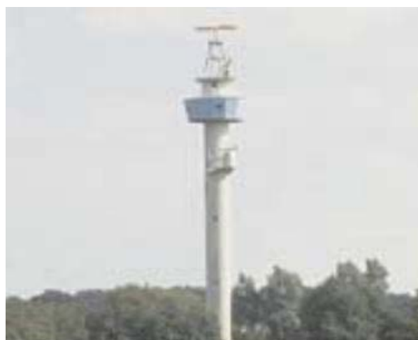
Tossens Radar Tower
