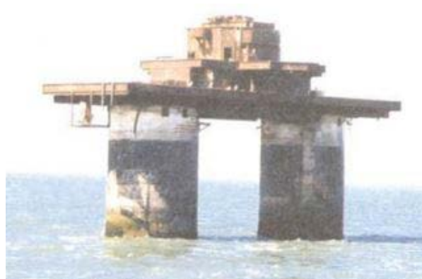
Knock John Tower
