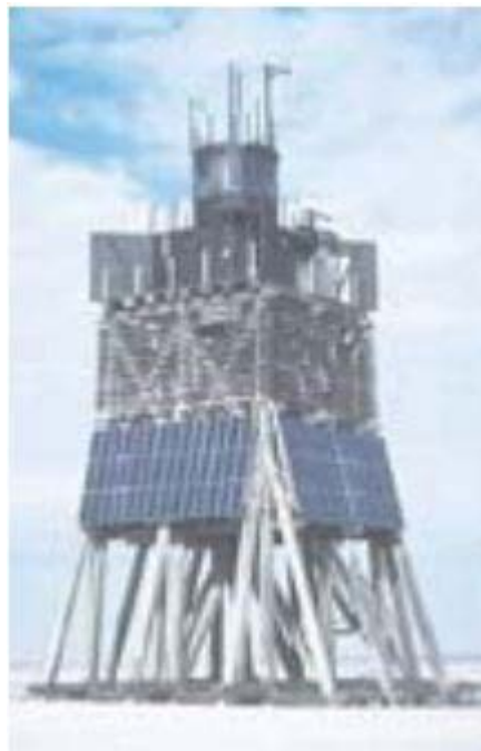
Suderoogsand Light (Refuge Beacon)
