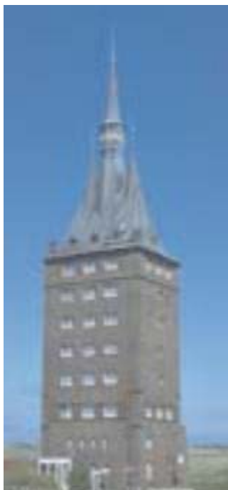
Wangerooge West Tower
