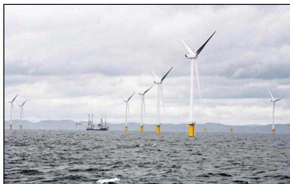
Humber Gateway Offshore Wind Farm Turbines
