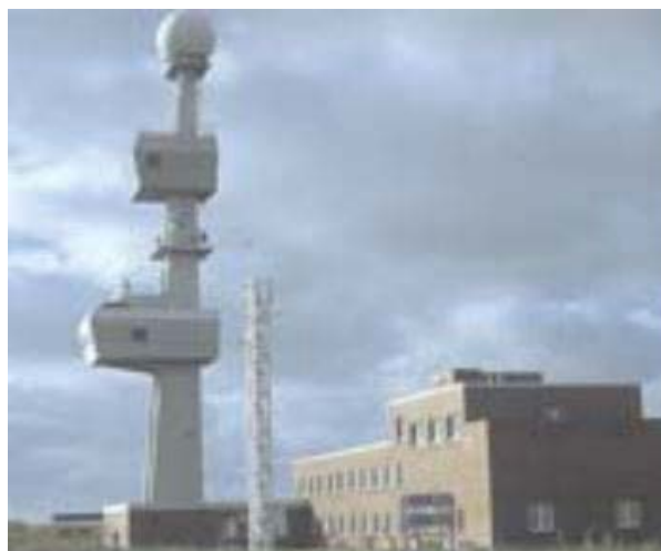
Knock Radar Tower (Light)
