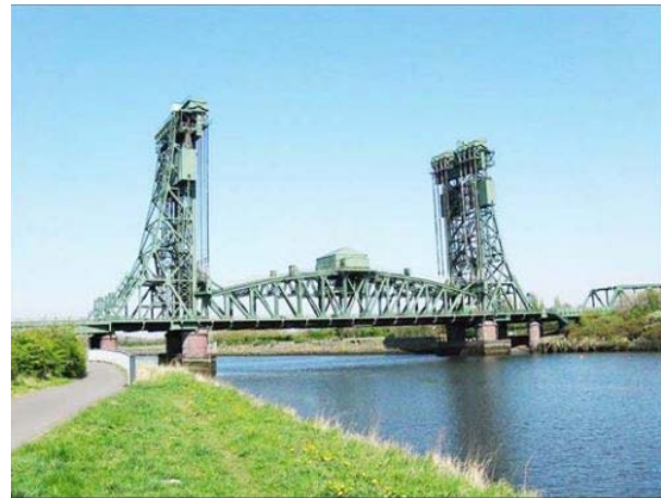
Tees Bridge (Newport Bridge)
