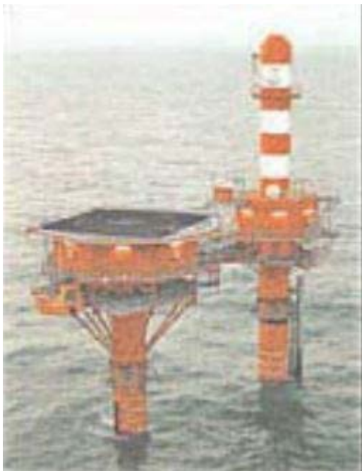
Oostdyck Radar Tower
