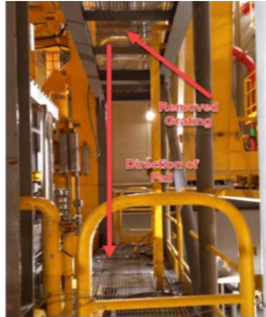
Hatch cover removed
